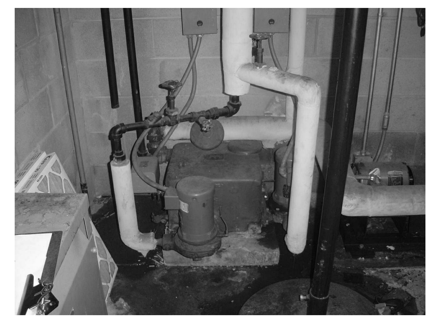
③ MECHANICAL ROOM CONDENSATE PUMP (CP-1) LOCATION 12" = 1'-0"
