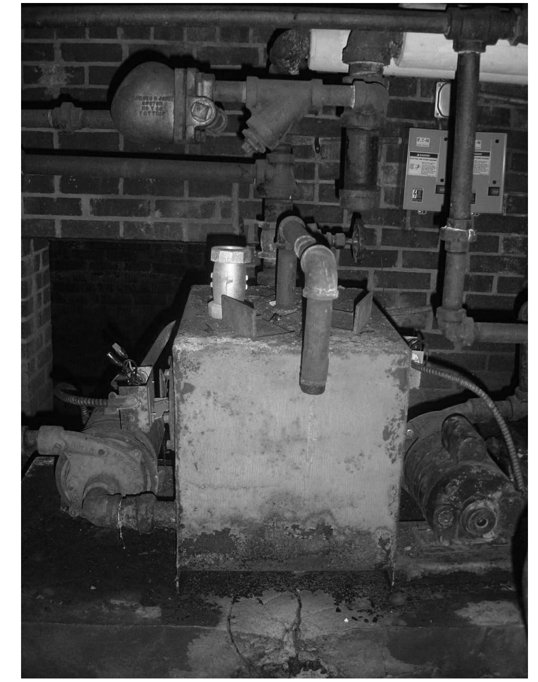
② CRAWL SPACE CONDENSATE PUMP (CP-1) LOCATION 12" = 1'-0"
